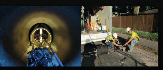
Elite Pipeline Services (EPS) is a provider of Joint Chemical Grouting Services. This joint grouting allows us to reduce or eliminate the infiltration of manholes and sewer lines, which is accomplished by sealing both the defect and the adjacent soil.
