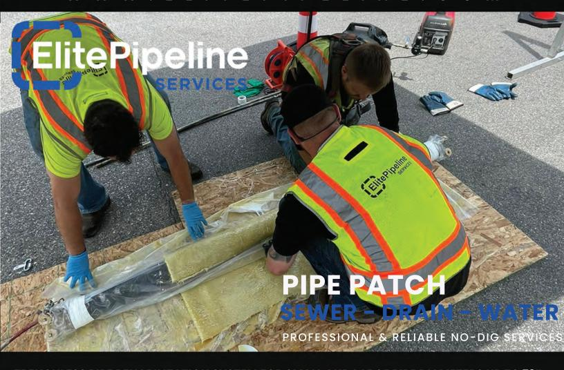
TRENCHLESS PIPE REHABILITATION SYSTEM FOR SMALL AND LARGE PIPE DIAMETERS UP TO 72"
