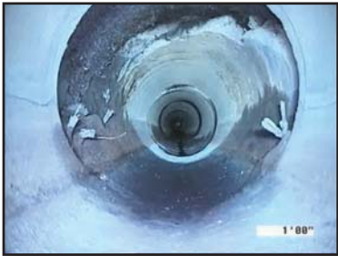
Concrete Loss
