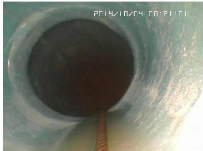
Pulling in a 6" to 4" Transitional Liner, Through a 2" Access Point.
