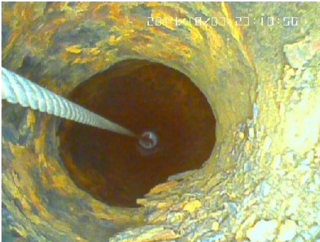
Pulling in a 6" to 4" Transitional Liner, Through a 2" Access Point.
