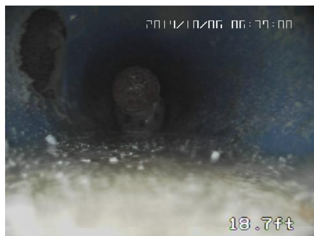
Reinstating Laterals from 100ft Away in a 4" Pipe Transition using a Robotic Cutter
