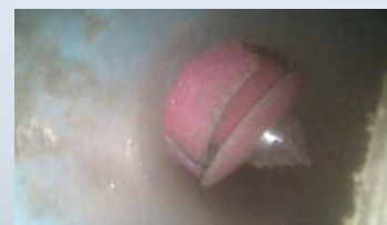
Pic 1. Reinstating through liner.
